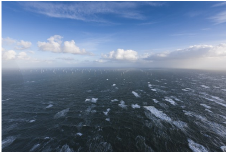
Figure 2.1 Example of wind mill farm in the North Sea that would have benefited from more accurate estimates of high frequent part of the wind sea spectrum
